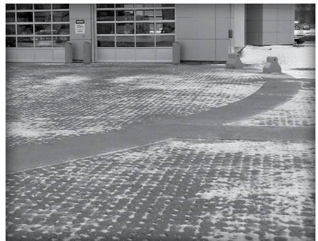
Figure 2. Examples of permeable interlocking concrete pavements for earning LEED® points. The photo on the left shows a hotel entrance in southern California. The photo on the right shows the driveway and parking lot for a fire station in Toronto.
