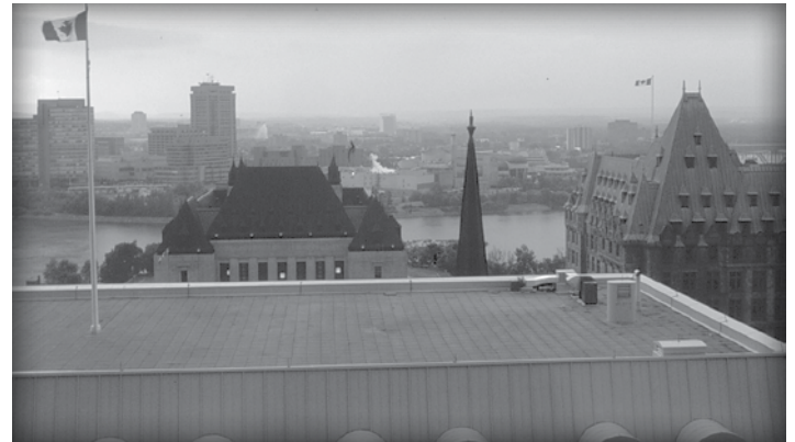
Figure 5. Light colored paving on low-slope roofs reflects light saving on air-conditioning costs while protecting the waterproofing.
